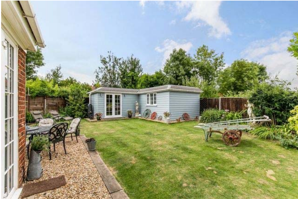
Figure 2: Outbuilding as built
